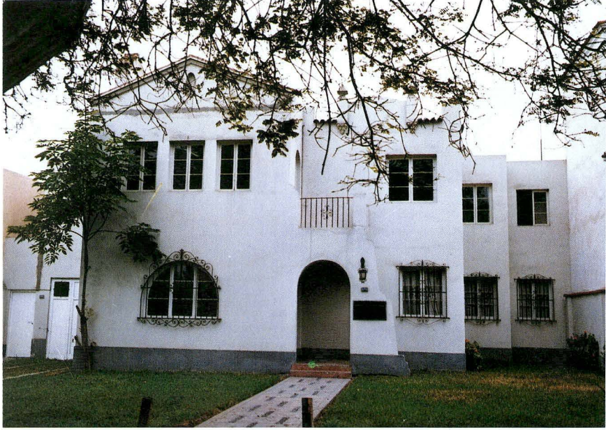
(7) Office for survey Team and Counterpart.
