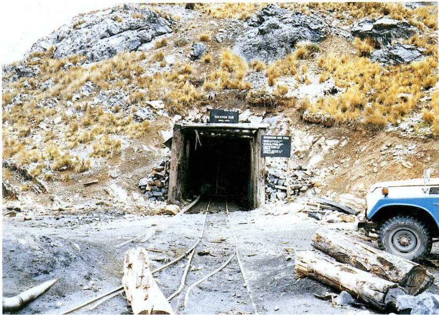
(14) Portal of S-adit (4,570 m above sea level).
