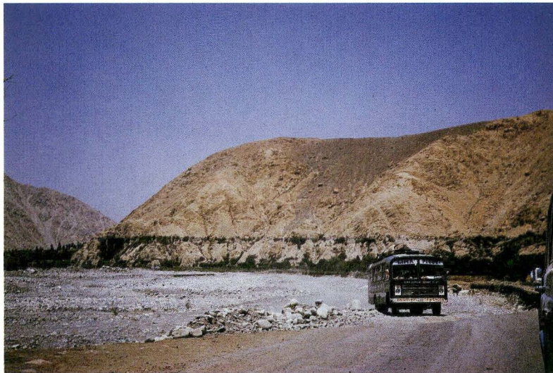
(10) Collapsed point of National Road No. 16 (12 km from Sayan).
